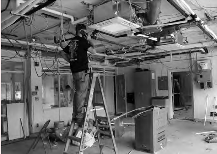
Infrastructure (such as electrical panels and wiring, ventilation, heat system piping, and more) has been updated. Work to update infrastructure items in the Main Office is currently underway, and is expected to be completed before students return in the fall.
