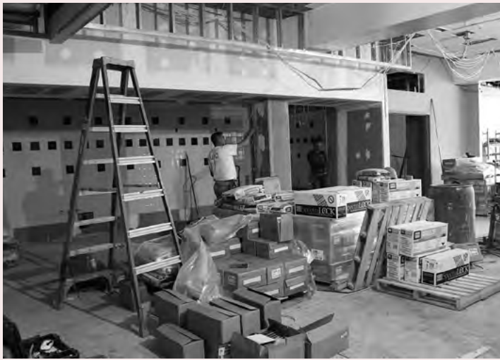
Work is underway to update the antiquated and undersized Central Kitchen. The kitchen renovation, the final part of the project, is anticipated to be completed by the time students return from Winter Break in January.
